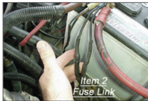
Also check the fuseable link that feeds the solenoid (Item 2) or fuse #9 in the fuse panel.
