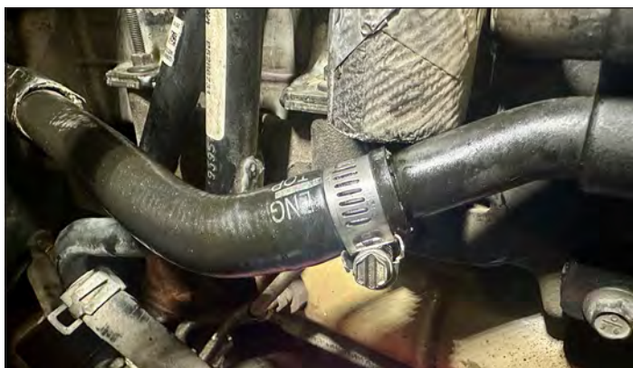
The OE spring-type hose clamp here gave me grief during reinstallation, so it was replaced with a common worm-gear clamp.
